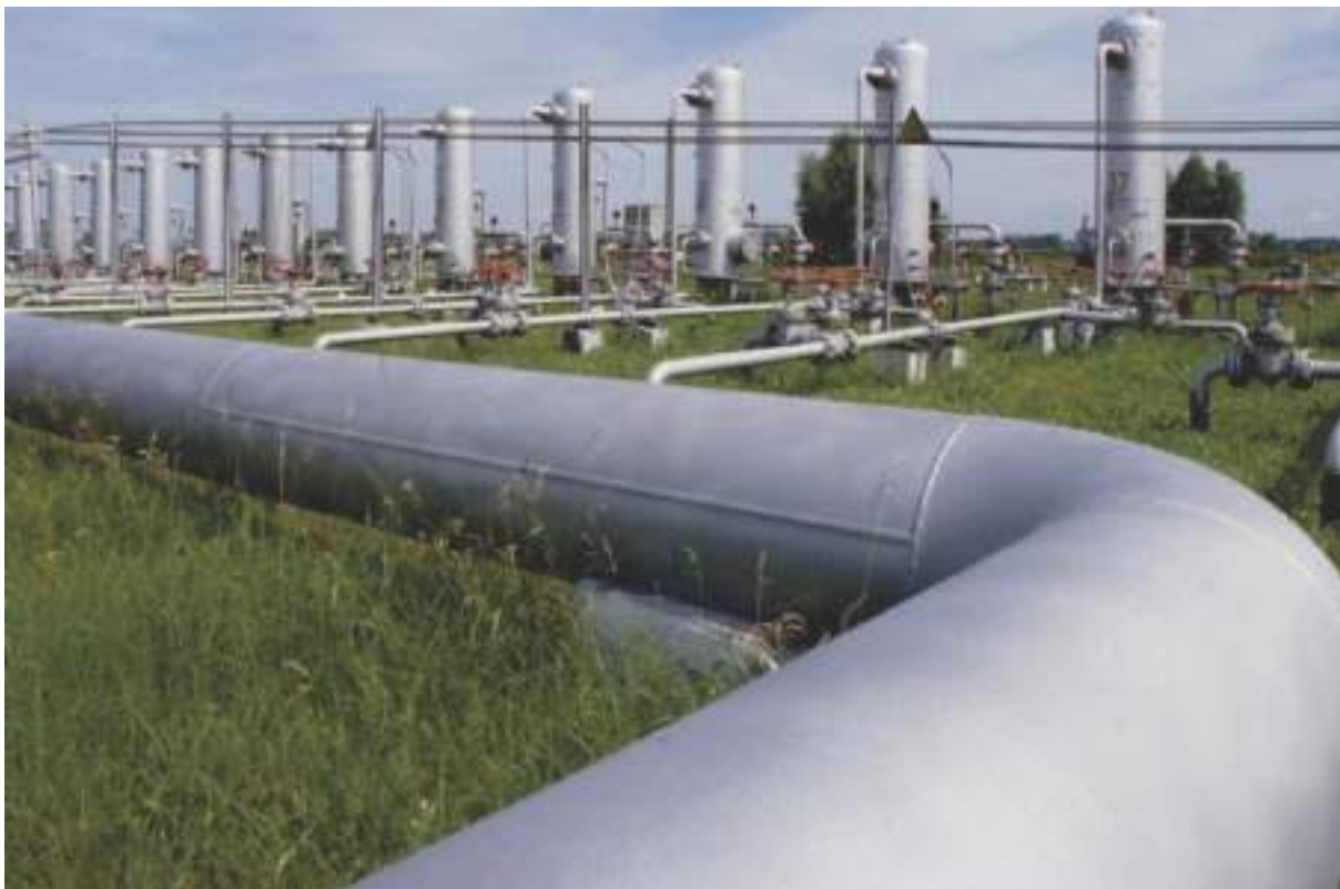
■ Oil Pipeline in Nigeria
