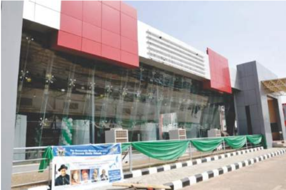
■ Re-modelling of Malam Aminu Kano International Airport in progress
