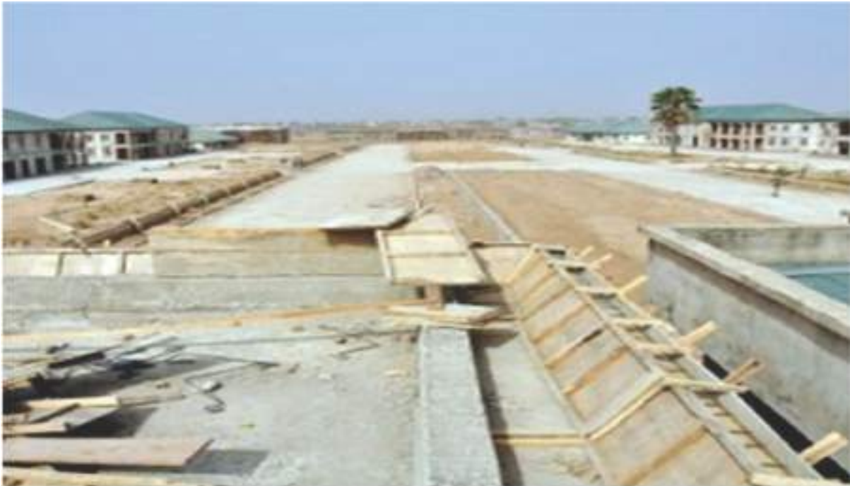
■ Construction works at Kashimbila Dam in Taraba State.
