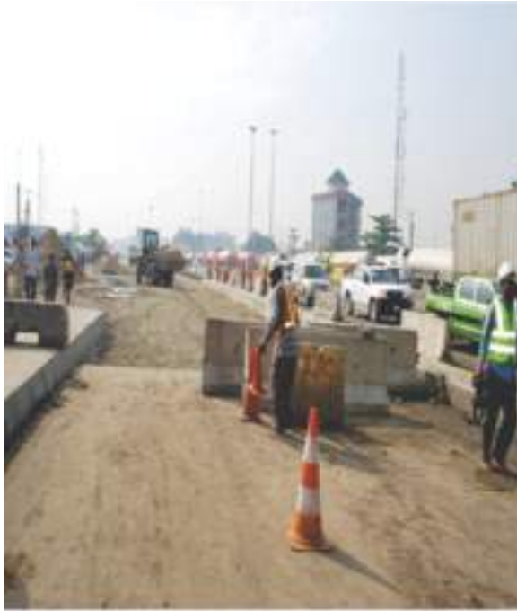
■ Road Rehabilitation work in progress
